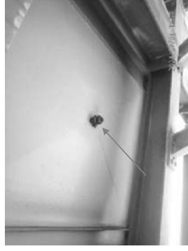
Drain port between pre and fine filter.
