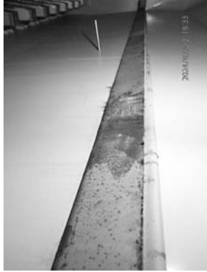
Corrosion condition found at the flexible joint area.
