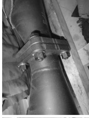
Big round pipe split line flange as found condition.
