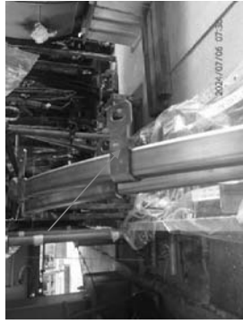
PT weld seal on big square pipe.
