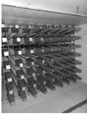
Silencer exit flow side seen from inlet casing side.
