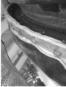
As found fabric bellow is good condition.
