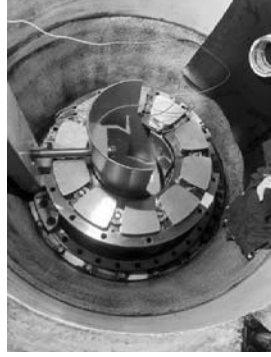
Installed new axial thrust pads during MP 60 inspection.
