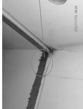
Example rusty observed inside inlet plenum at connecting joint duct between silencer and plenum.
