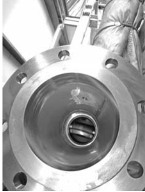
Butterfly valve condition inside the pipe.
