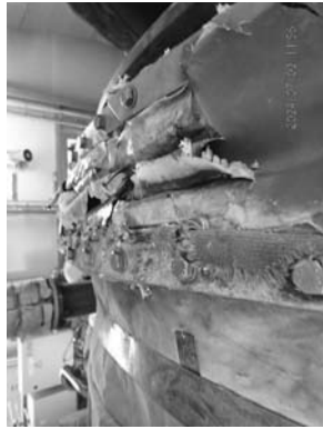
Example view on fabric bellow condition.
