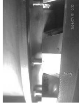
New rotor tie nuts were replaced during this outage.
