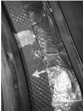
Example view for condition on Insulation cassette from previous repaired at cassette no. 3,4 (clockwise).
