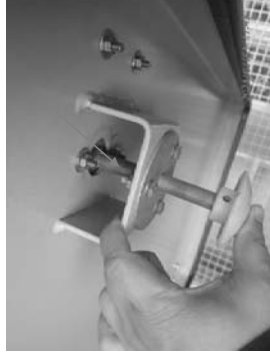
Emergency door release was in good condition.
