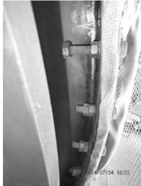
Outlet casing overall condition before dismantling. Observed double nuts missing and loose around fabric bellow.
