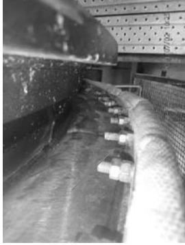
The outlet bellow bolts were good condition.
