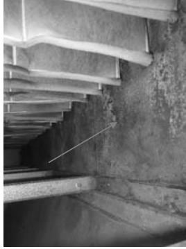
Ventilation filter housing floor condition.
