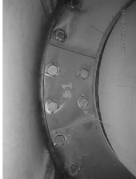
Example central seal segments before dismantling, no bolts damage.
