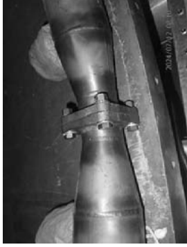
Replaced new gasket on big roll pipe.
