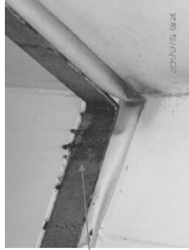
Example rusty observed inside inlet plenum at connecting joint duct between silencer and plenum.
