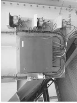
Intake filter housing instrument panel condition.
