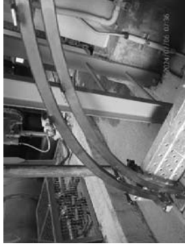
Support square brackets were broken.
