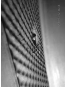
Insulation cassettes damaged at position 6.
