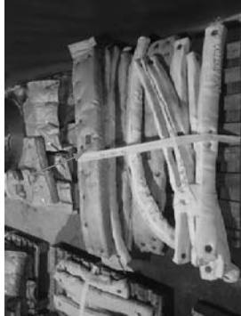
Example of insulation as found condition.
