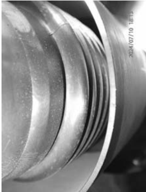
Example of minor deformed on outlet bellow condition.
