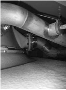
Lube oil supply line and return line at bearing 1.
