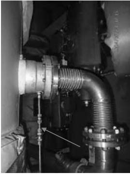
Jacking oil check valve to bearing 2 condition.
